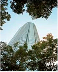
Roppongi Hills Mori Tower, Tokyo
